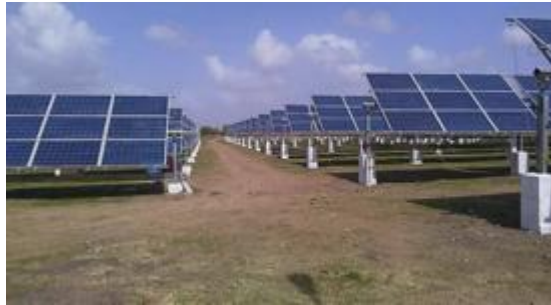
Poly Crystalline 0.5MW Kutch, Gujarat Completed 2015
